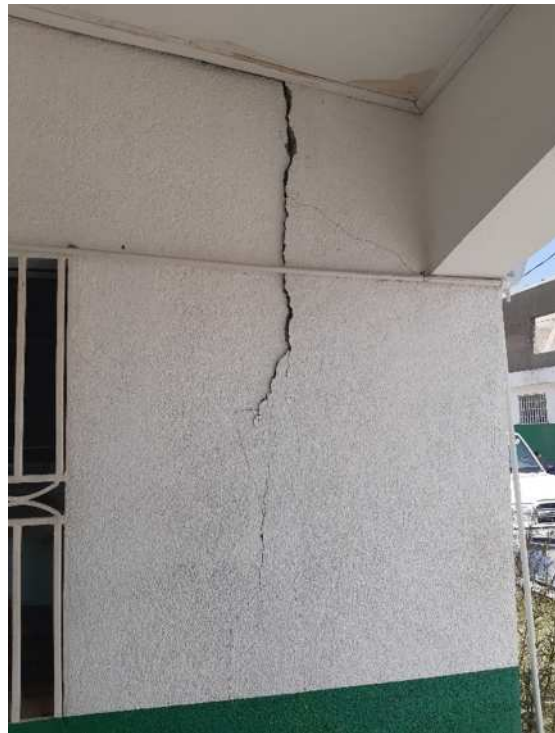
Figure 27 - Crack on the supporting structure of the portico
