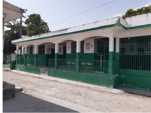
Figure 26 - Area of building 13 that could not be accessed
