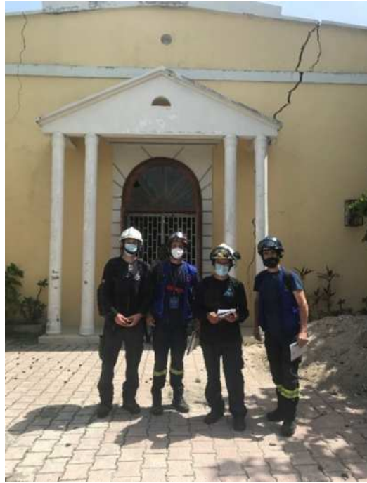
Figure 38 – Building 22 structural cracking visible at the East facade
