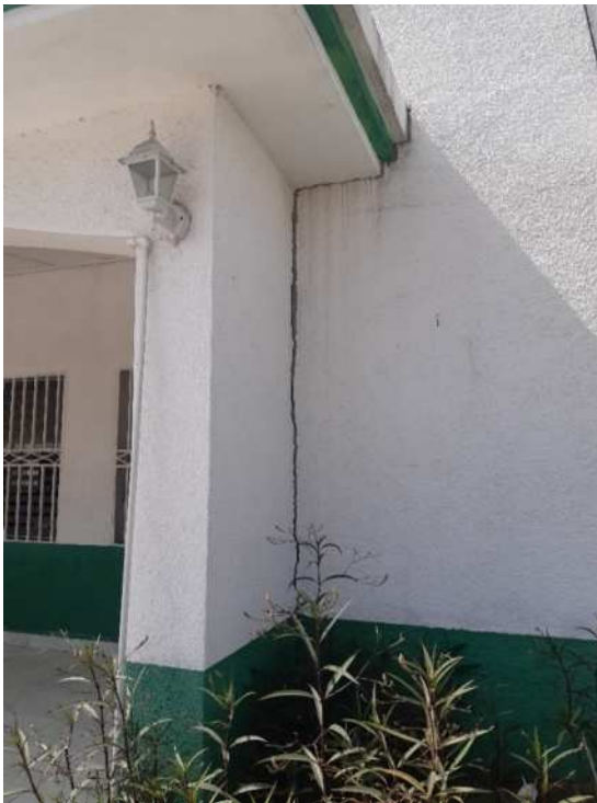
Figure 27 - Crack on the supporting structure of the portico
