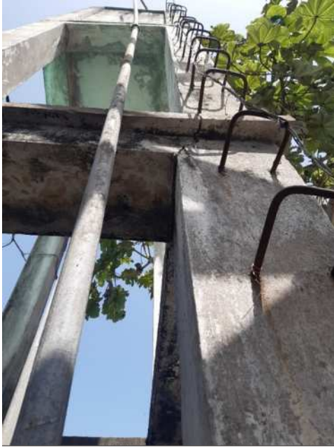
Figure 8 - Building 3, concrete water tower
