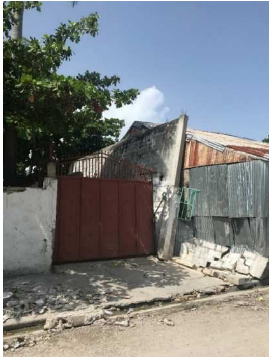
Figure 42- Building 25 boundary wall
