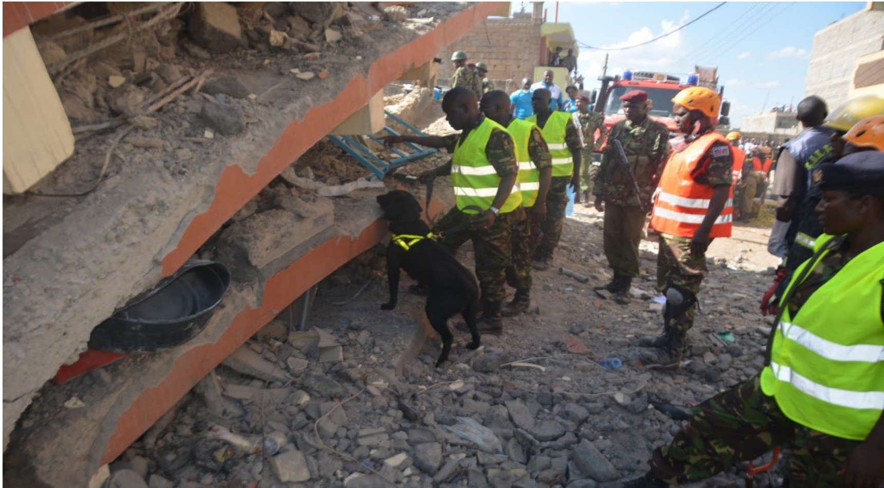
Tassia collapsed building 8 TH DEC 2019
