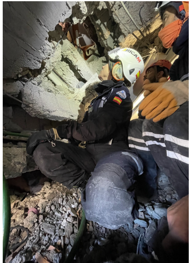
USAR operations inside of a damaged building
